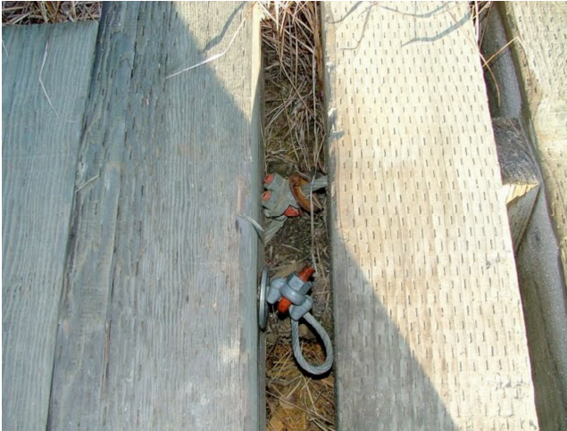
Figure 5 As-built image of one side of the cable clamped ATV boardwalk at CPCRW.
